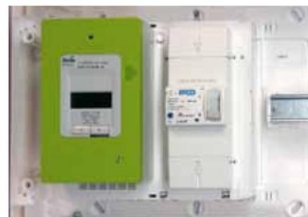
Up to 4 modules can be added to this electrical box, on the modular rail.
