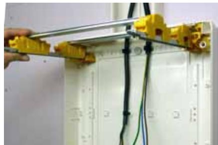
The chassis can be pulled out completely to make it easier to fix the cabinet in place, or to install and wire up equipment on a work surface.
