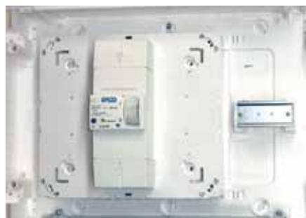
Electrical box Cat.No 4 016 53 is used to connect a subscriber MCB and a CBE or LINKY single-phase electronic meter. This cabinet is supplied with plate Cat.No 4 011 81, on which the “blue tariff” circuit-breaker is fixed.
