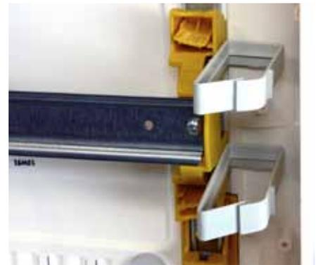
XL<sup>3</sup> 125 cabinets can accommodate LINA 25 cable ducting with maximum dimensions of 40 x 60 mm (Cat.No 0 362 07).
