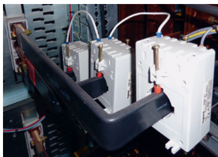
Current transformers mounted directly on flexible busbars
