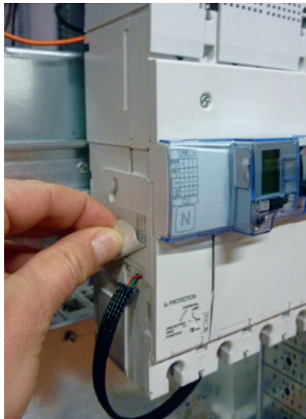
Connection on the left-hand side of the DPX 3 , under the label.
