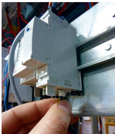
Connection under the communication interface. The connecting cable is supplied with the interface.
